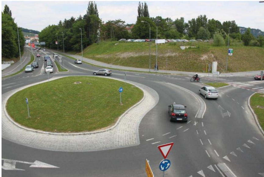
Fig. 5. Typical Slovenian turbo-roundabout (with divided curbs)
