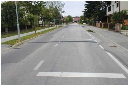
*Fig. 1. Optical breaks (rumble strips) before intersection (Murska Sobota)*
